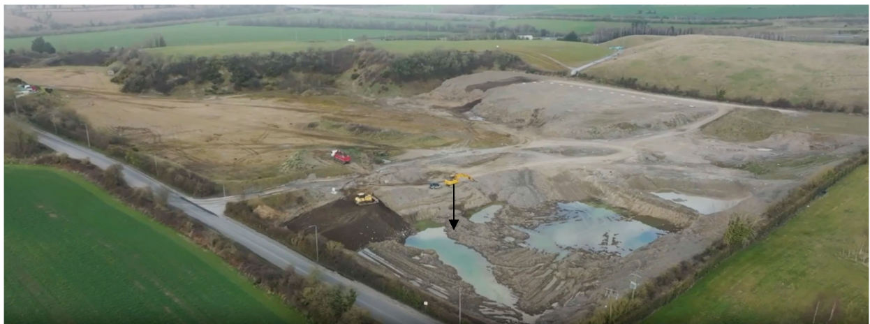
View from southeast (active quarrying in foreground)
